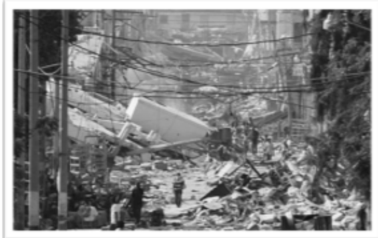
Figure 1. Damage after the 2010 earthquake in Port-au-Prince, Haiti.
