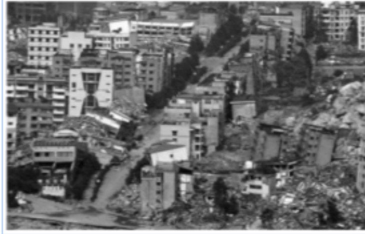
Figure 1. Damage after the 2008 earthquake in Sichuan, China.
